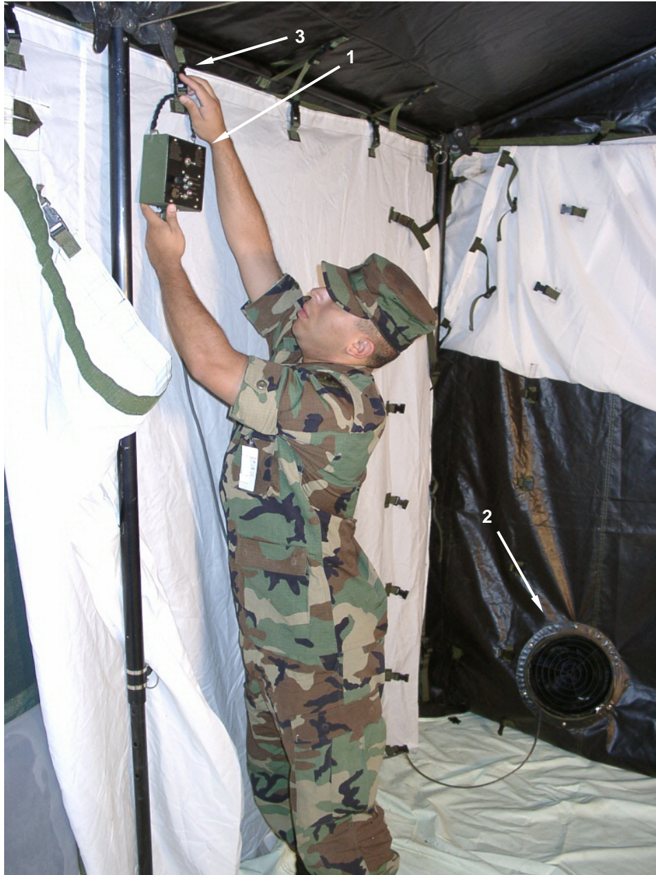
Figure 17. Positioning the In-tent Controller Inside the Tent.
