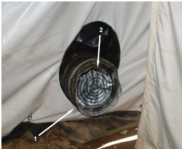
Figure 1. Return and Supply Ducts.
